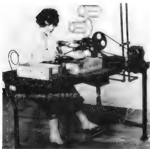
Hand-operated 2-head flange machine as used by Westinghouse in 1914.
